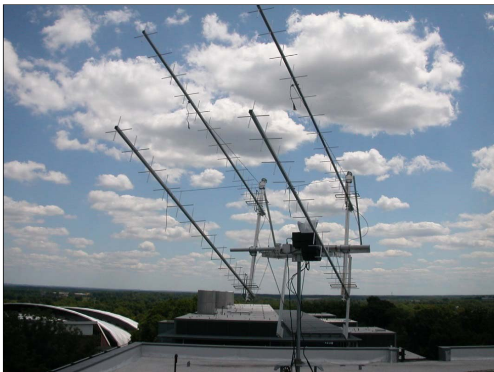
Fig. 1: Four-Yagi dual-polarization 432 MHz array at W2PU. The Yagis are rear-mounted; boom length is 3.5 m, and stacking distance is 1.2 m in each direction.
